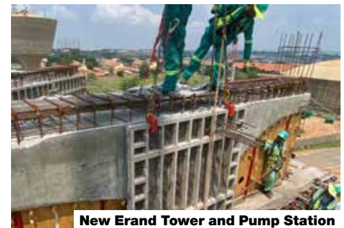
New Erand Tower and Pump Station
