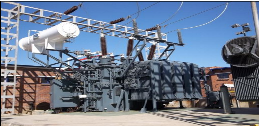
Figure 12 Substation upgrades and installations in Robertsham
