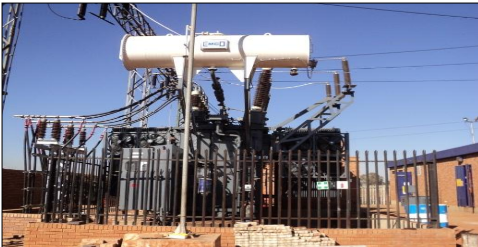
Figure 15 Nancefield substation upgrades and installations
