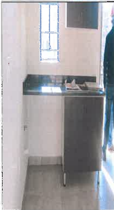
Devland Project: Finishes
