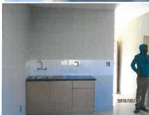
Dobsonville Project: Finishes
