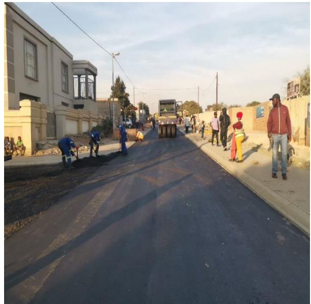
Images 11 & 12: Upgrading of Gravel Roads and stormwater in Diepsloot
