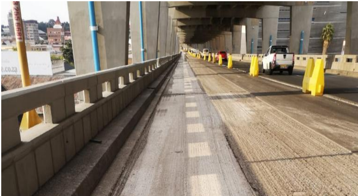
Image 13: M1 Double Decker rehabilitation
