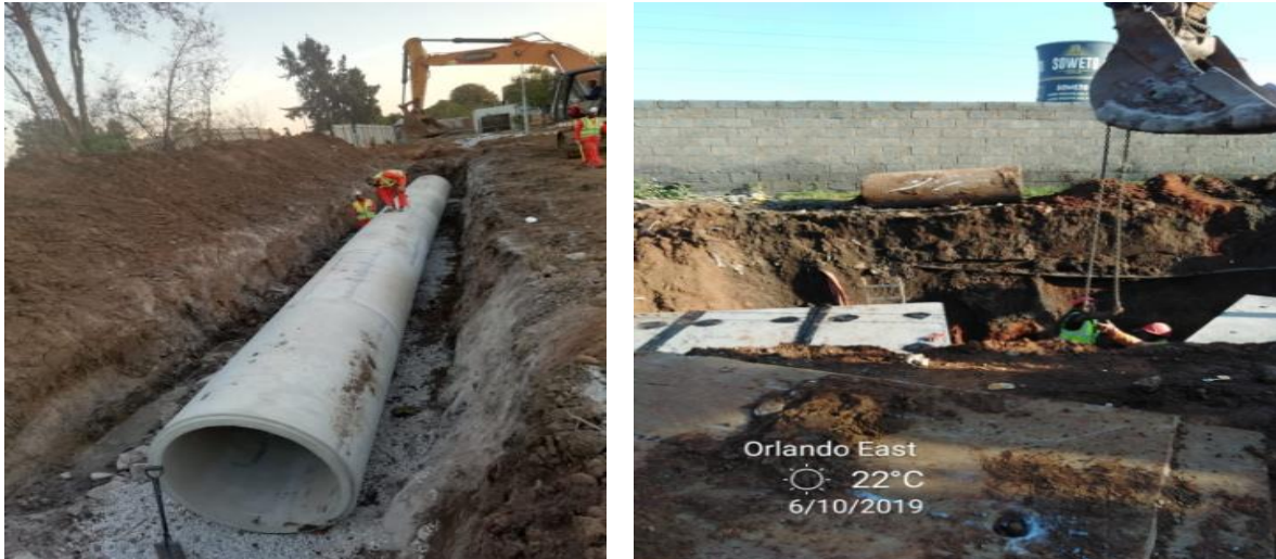
Images 20 & 21: Implementation of the Stormwater Master Plan in Soweto
