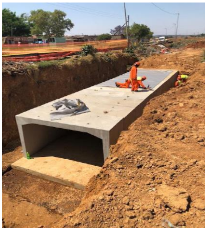
Images 18 & 19: Conversion of Open drains into closed system in Orange Farm and Ivory Park
