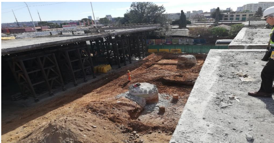
Image 14: M2 Selby deck demolition
