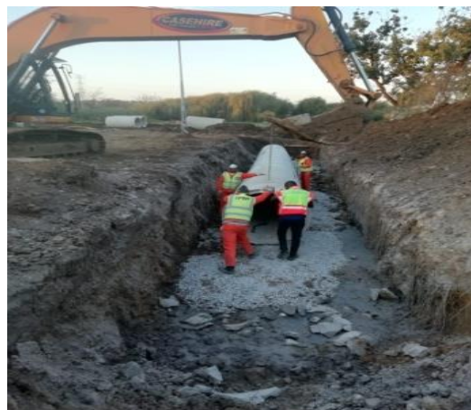
Images 18 & 19: Conversion of Open drains into closed system in Orange Farm and Ivory Park
